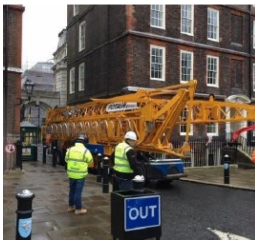
Crane arriving on site on 15 February
