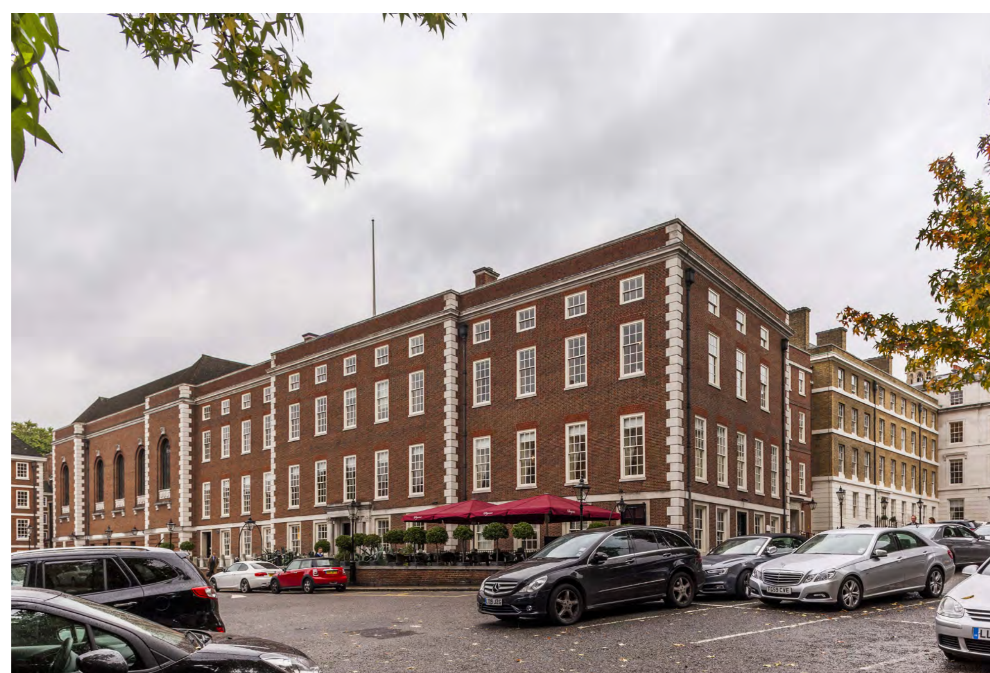
Existing View from Inner Temple Car Park
