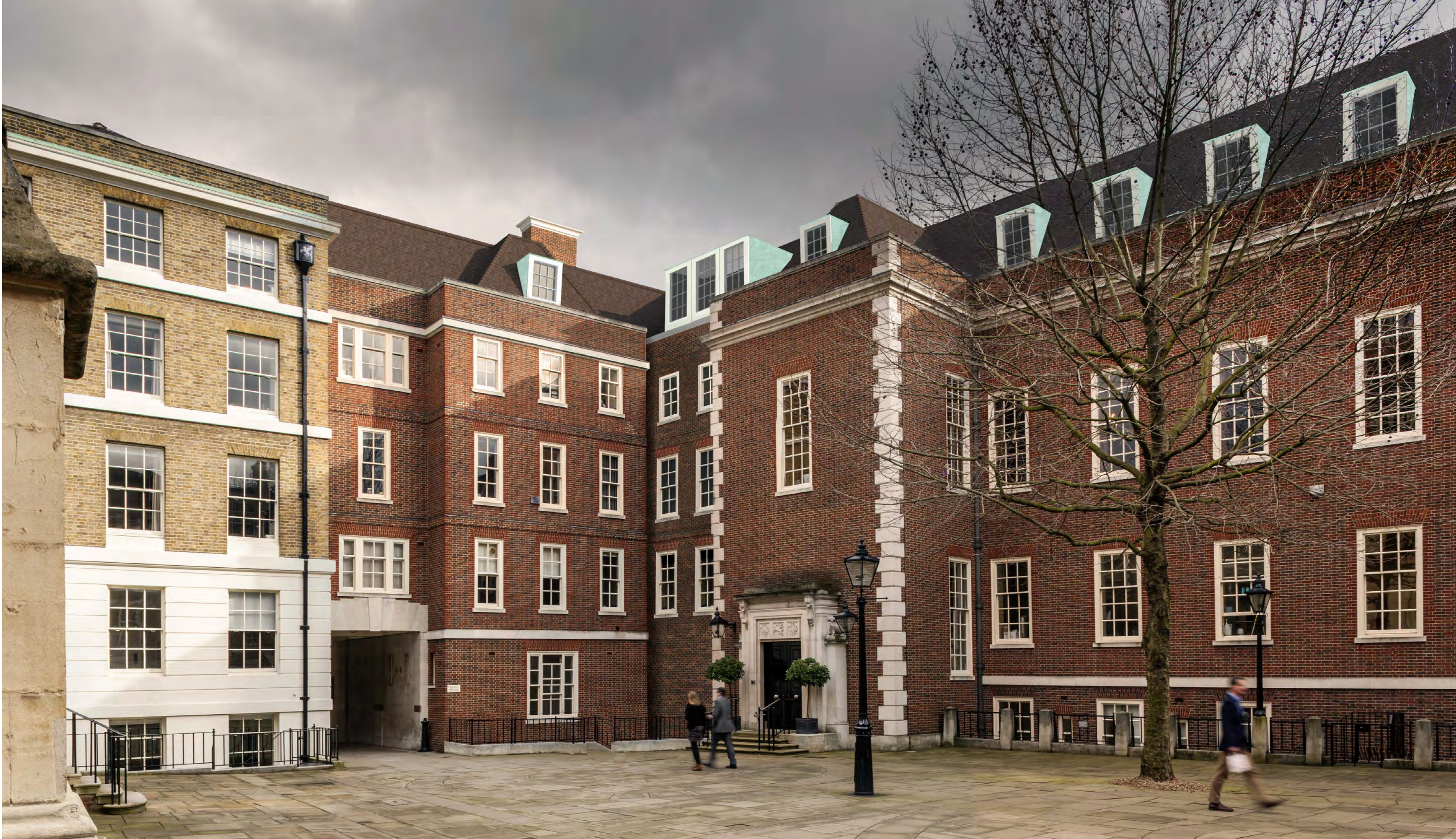
Proposed view from Church Court. A new lift core is proposed adjacent to the Benchers' Entrance, designed in matching brickwork with stone detailing and sash windows
