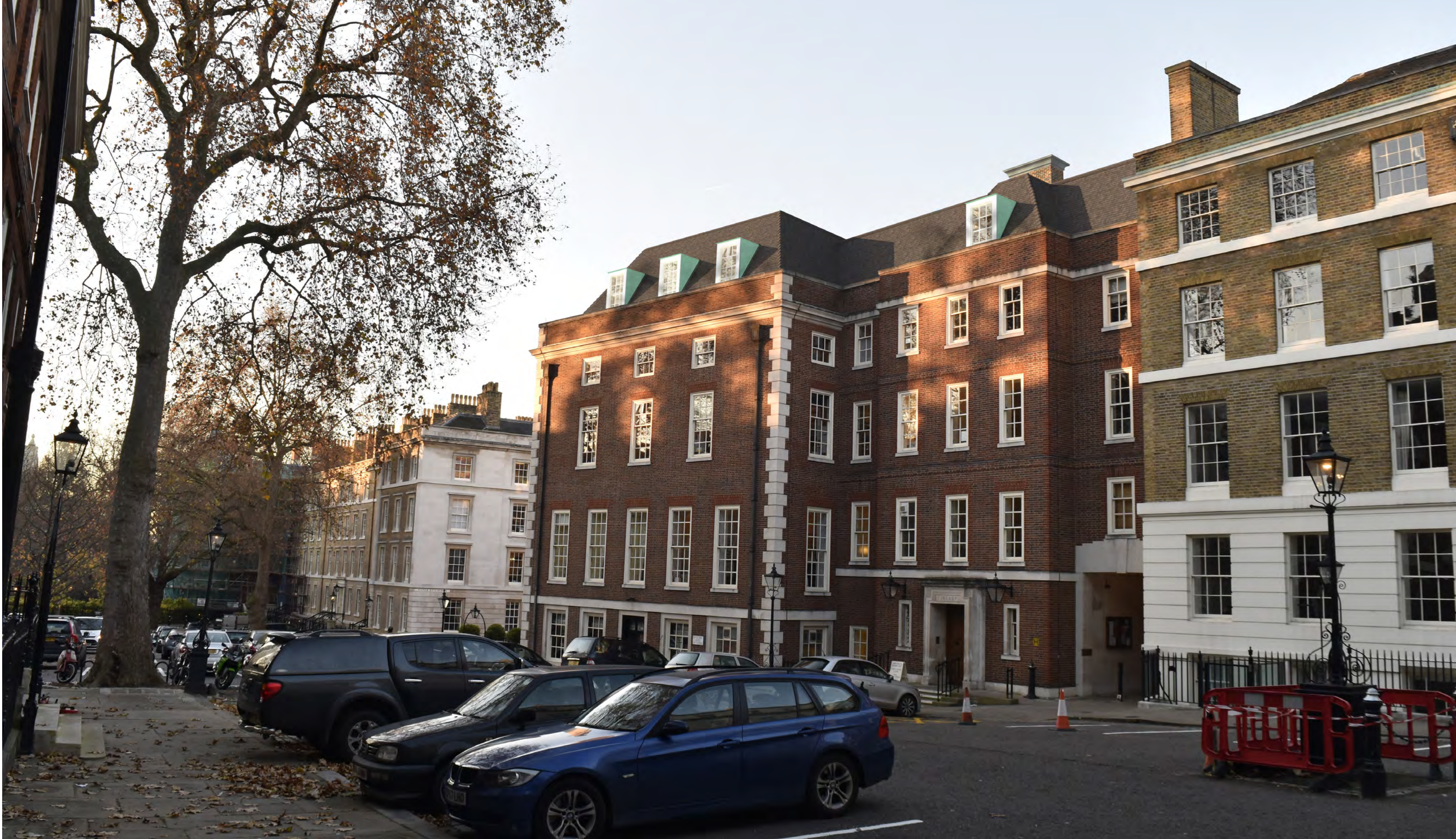
Proposed view from King's Bench Walk showing the new Education and Training Centre contained with a clay tiled mansard roof extension
